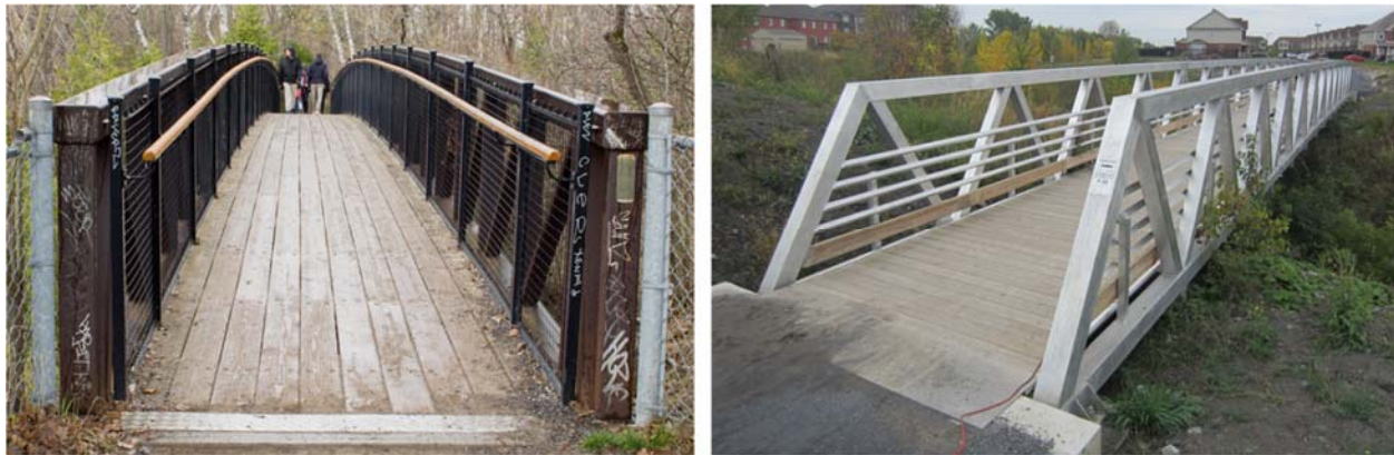
Figure 1: Typical steel (left) and aluminum (right) pony truss pedestrian bridges.
