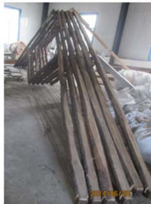
(b) A picture of the wood-steel roof trusses
