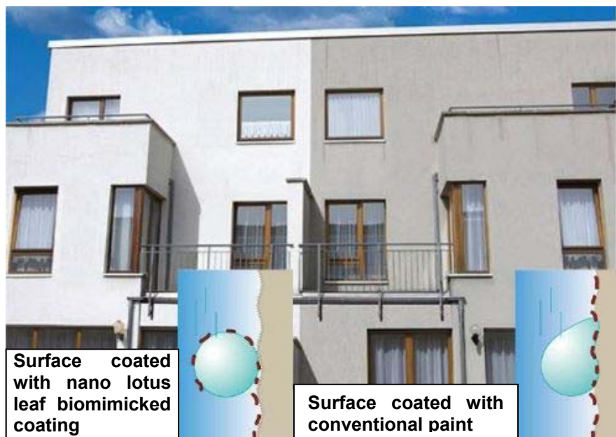
Figure 6: Comparison of conventional and nano lotus leaf biomimicked coating (adapted from European Consumers Choice 2017)
