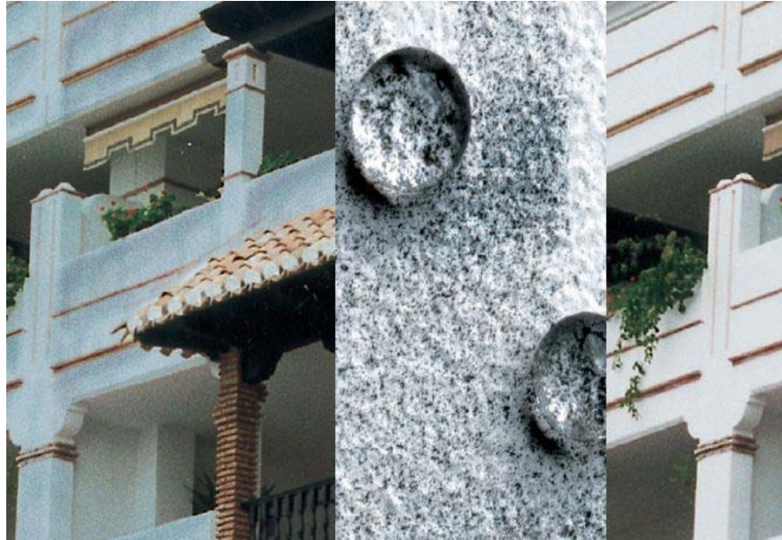
Figure 5: Application of nano lotus leaf biomimicked coating and its effect on the facade of a building (adapted from Sto Corporation 2017)
