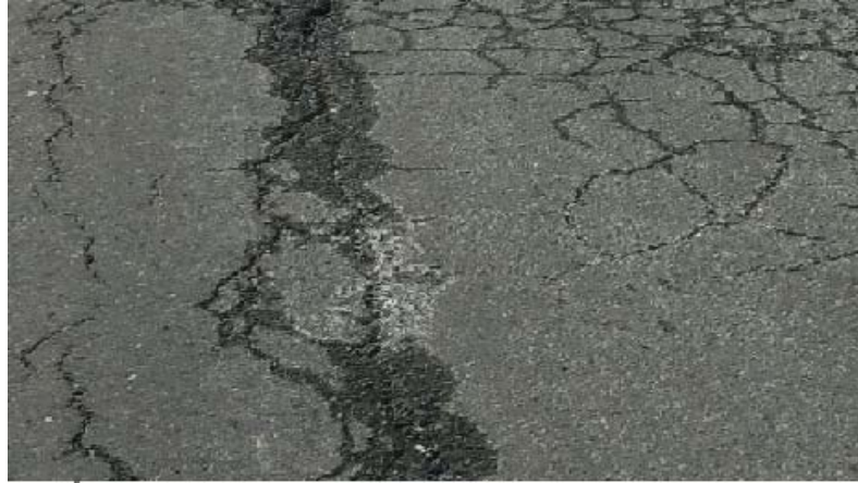
Figure 4: Block cracking
