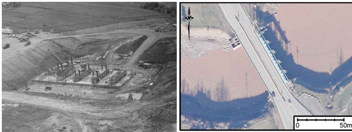
a) During construction June 29, 1966
