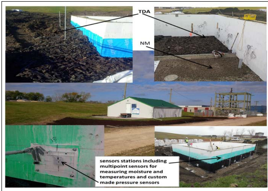
Figure 1: The Experimental House at RRC
