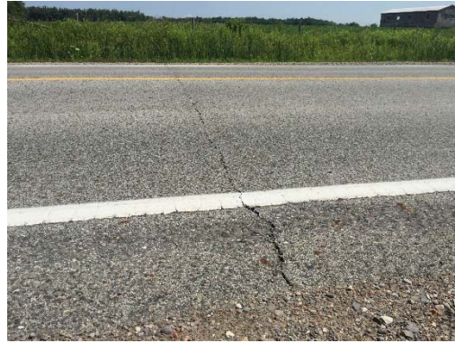
Transverse Cracking
