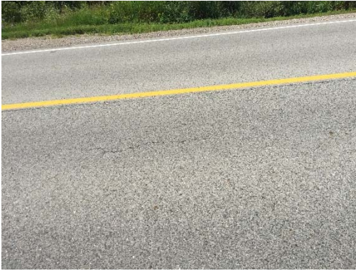
Minor crack
