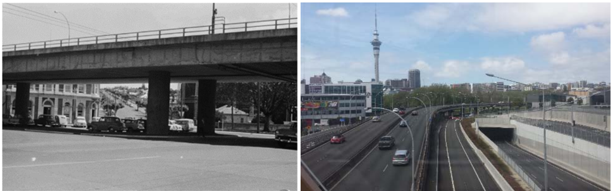
Figure 3: 1962 View of VPV and ASR Cracks (left), View of VPV and VPT looking South (right)
