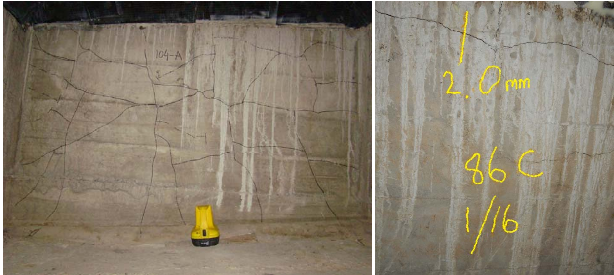
Figure 6: Example of Condition Inside Box Cells
