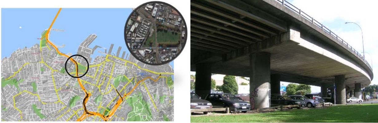
Figure 2: Location Map (left), Elevation Photo of North VPV Box Structure (right)
