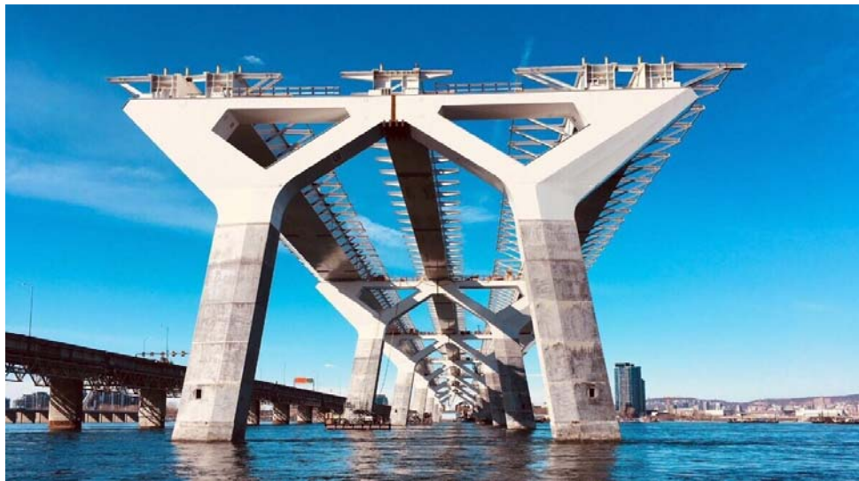
Figure 1: Construction of the new Champlain Bridge, Montreal
