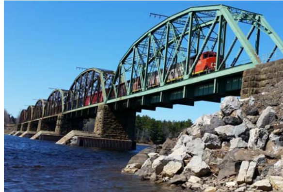
Figure 2: Photo of the bridge looking downstream from the south approach embankment.
