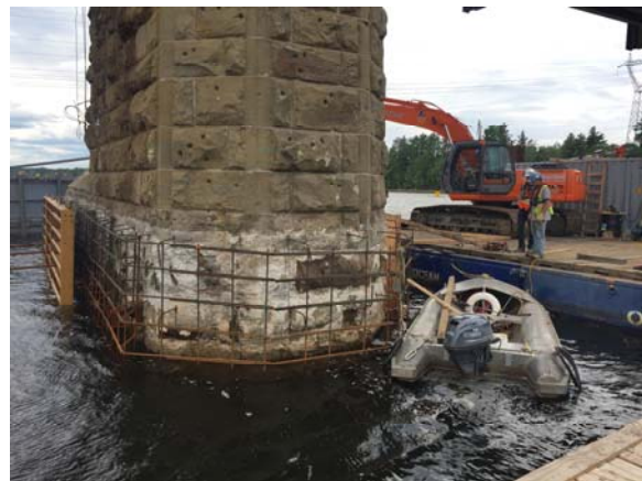
Figure 8: Repair work in 2017.
