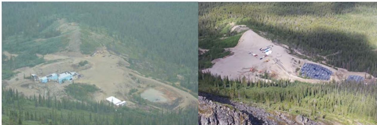
Figure 1: Site photo (left, 2010) taken prior to remedial activities; mill building left and tailings pond right. Site photo (right, 2017) taken during remedial activities; mill building demolished, site capped and liner being installed on tailings and sedimentation ponds.
