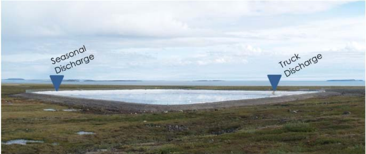
Figure 1: Kugluktuk sewage lagoon with white HDPE liner.
