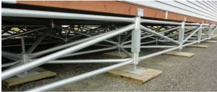
Figure 4: Lattice structure under northern home
