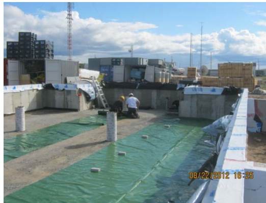
Figure 3: Building Basement in the North
