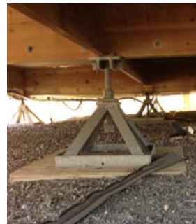
Figure 2: Steel footing under steel beam.
