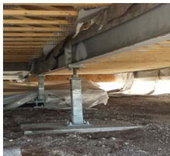
Figure. 1: Steel tripod footing.
