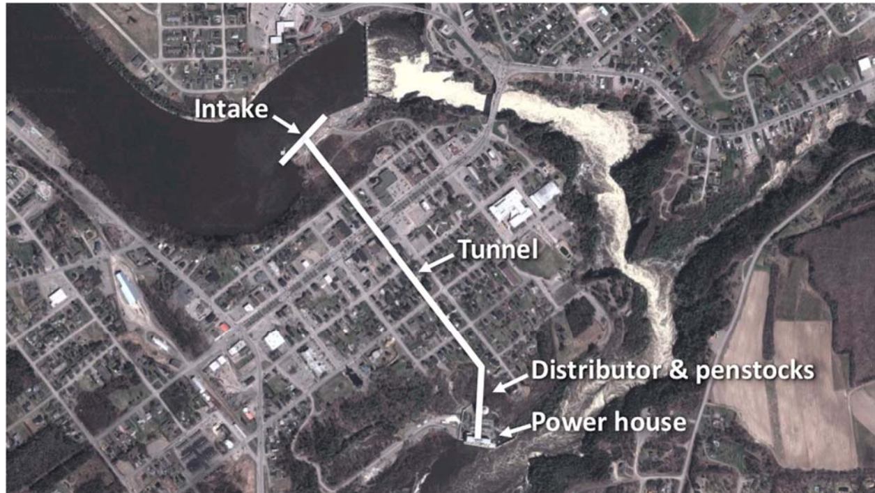
Figure 1: Sketch of the Grand Falls Generating Station intake tunnel
