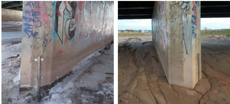
Figure 3 Sediment Accumulation Bay of Fundy at Tide Gauge Location (March 2013 Left, January 2014 Right). Credit: Alexander Wilson, CBCL Limited
