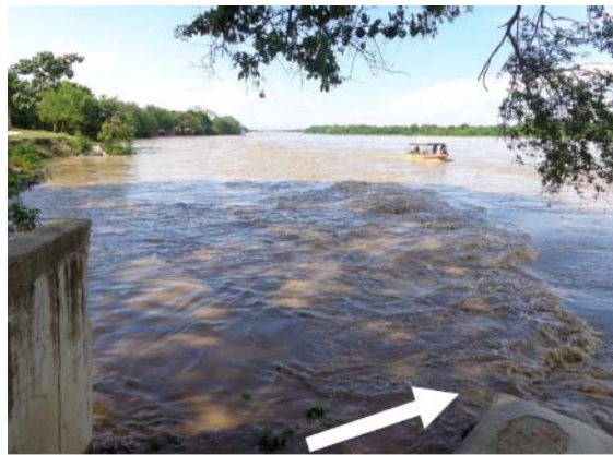
Figure 5. Ripples observed in front of the retaining wall, “El Conejo” neighborhood (Vargas July 2017).
