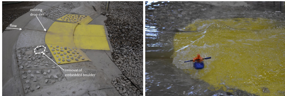
Figure 2: Side view looking at the recommended design of the rehabilitation of HWC Drop #4 (left) and the wave forming on this drop at a river discharge of 150 m 3 /s (right).
