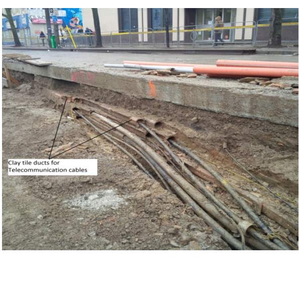
Figure 6: Clay tile ducts structure
