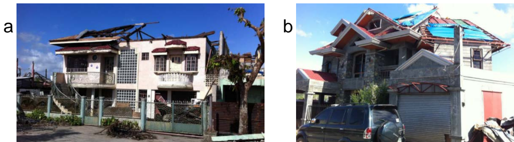
Figure 12. Example (a) older construction, and (b) newer construction.
