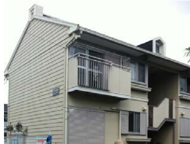
Figure 11. Example of residential building in Japan with all glass windows (and doors) having shutters that can be closed shut to add protection during a wind storm.
