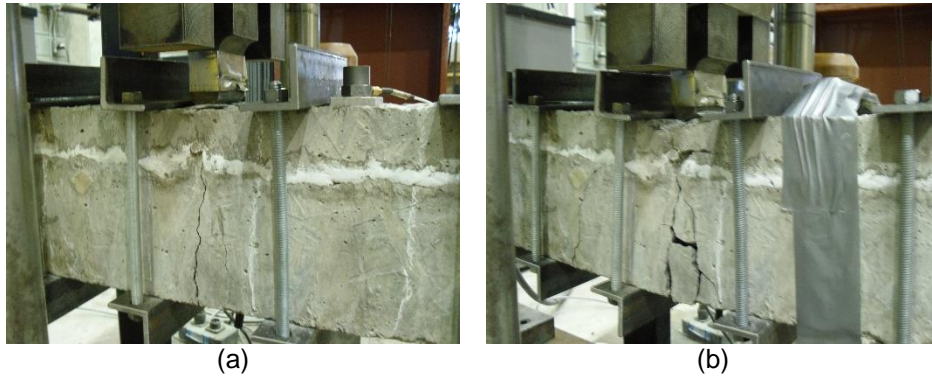
Figure 5: Post-test photos of Beam 1 (Control): (a) post 175-mm (b) post 200-mm drop
