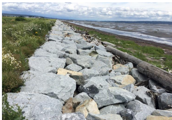
Figure 9: Upgraded section of dike at Boundary Bay (2015)
