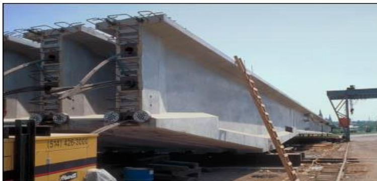
Figure 2: View of a CPCI I Girder (Retrieved from http://www.cpci.ca )
