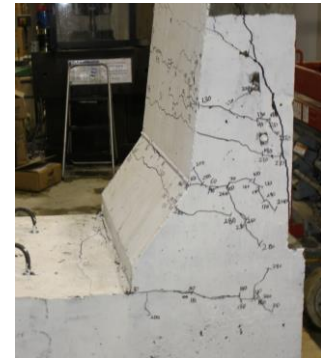
Figure 20: Cracks on right side of B-5
