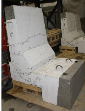
Figure 8: Crack pattern on the left side of B-1
