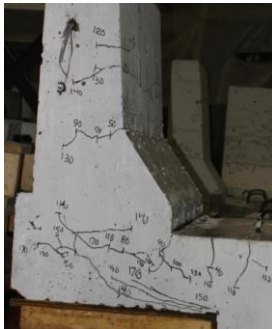
Figure 15: Cracks on left side of B-3
