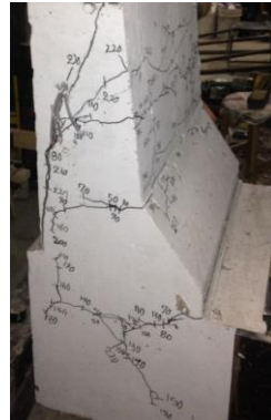
Figure 19: Cracks on left side of B-4
