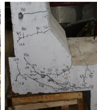
Figure 12: Crack pattern in the left side of B-2
