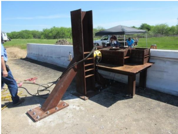
Figure 11: View of the test setup at for static load test at interior location
