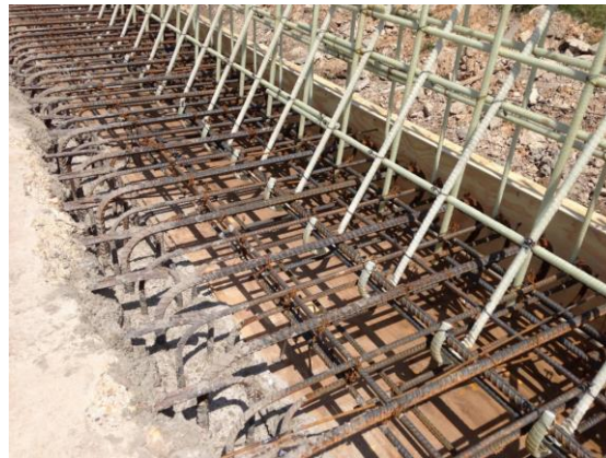
Figure 6: Close-up view of the hooked GFRP bars and deck
