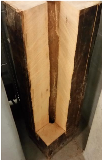
Figure 8. A heritage Beam (no. 3) after two strips were cut out to be tested under a controlled heat exposure. Note the hollowed core was traditionally added to prevent moisture accumulation.
