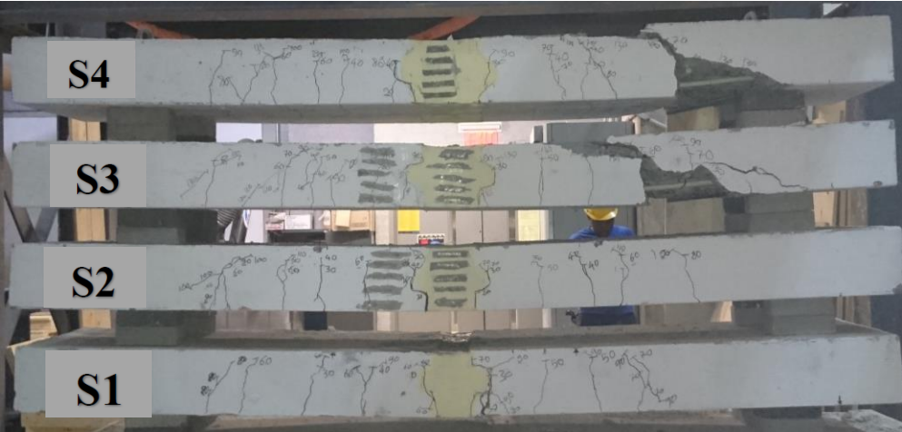
Figure 5: View of failure modes of the slabs from side 2
