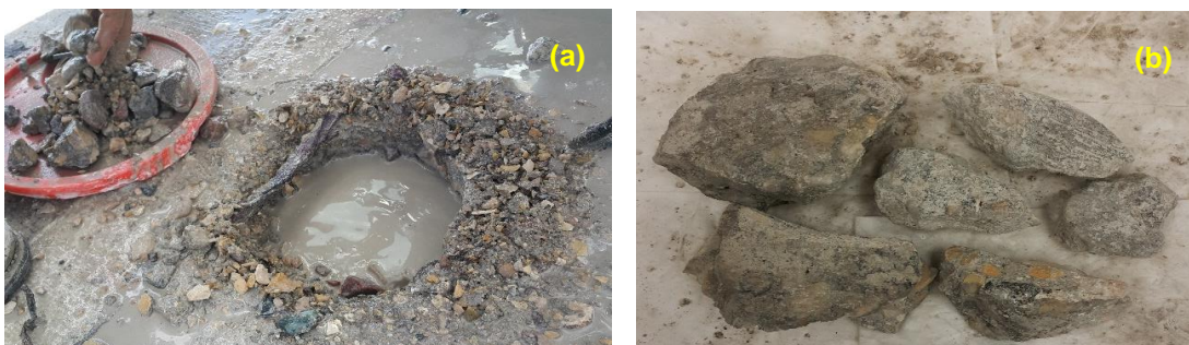
Figure 2: An example from regional roads showing: (a) damage of concrete during the coring process, and (b) fractured core.
