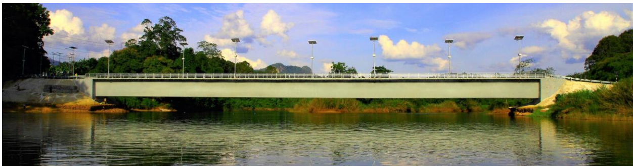
Figure 9: UHPC Box-Girder Bridge – Batu 6 Bridge over the Perak River, Malaysia
