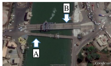
[b] Old and New Azmy Bridges
