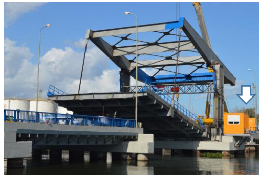
Figure 7: view of the bridge during opening, showing operation Service operating room
