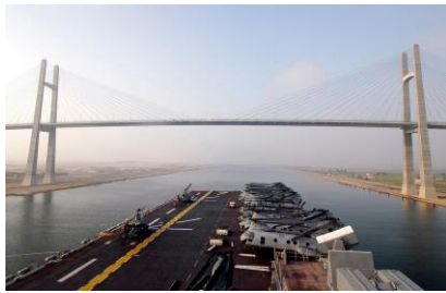
[a] Cable stayed bridge
