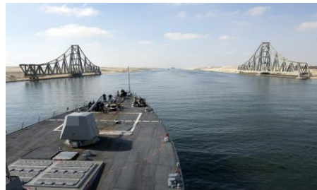
[b] Al Ferdan swing bridge
