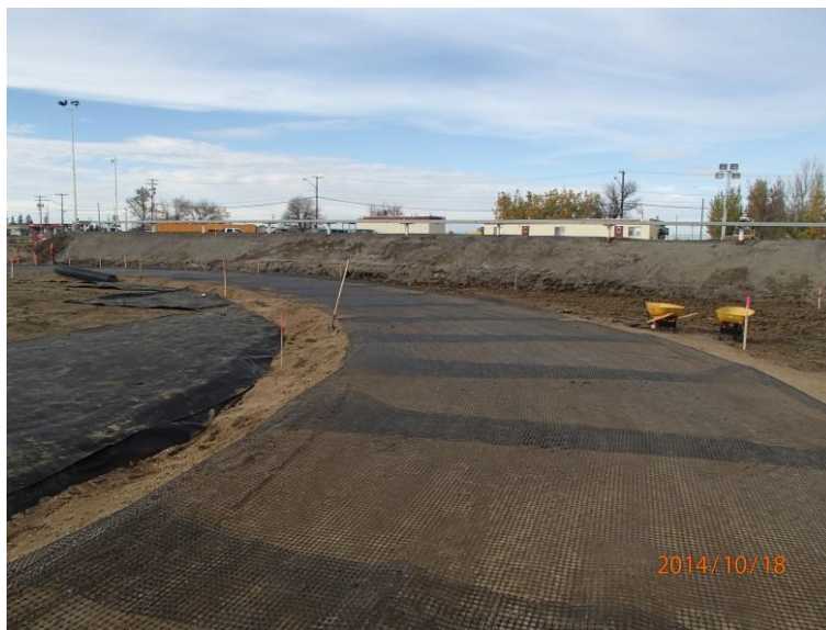
Figure 4 – Biaxial Geogrid Placed above Installed Geosynthetic Cellular Confining System (GCCS)
