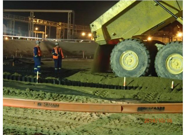
Figure 3 – Placing Gravel within Geosynthetic Cellular Confining System
