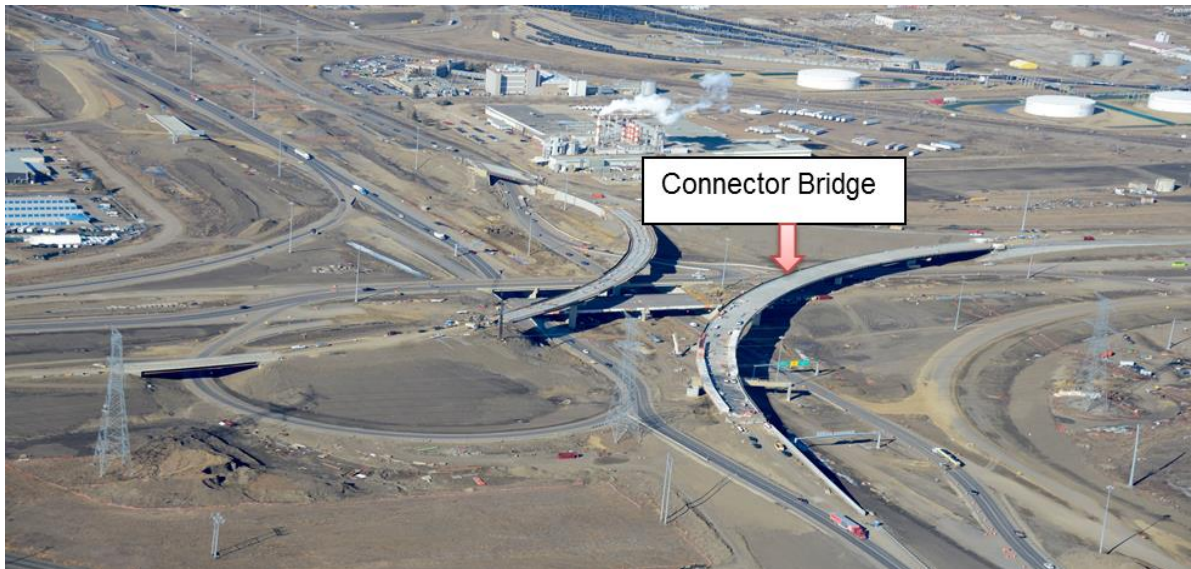
Figure 6: Completed Connector Bridge Structure Between the South Bound Anthony Henday and East Bound Yellowhead Highway
