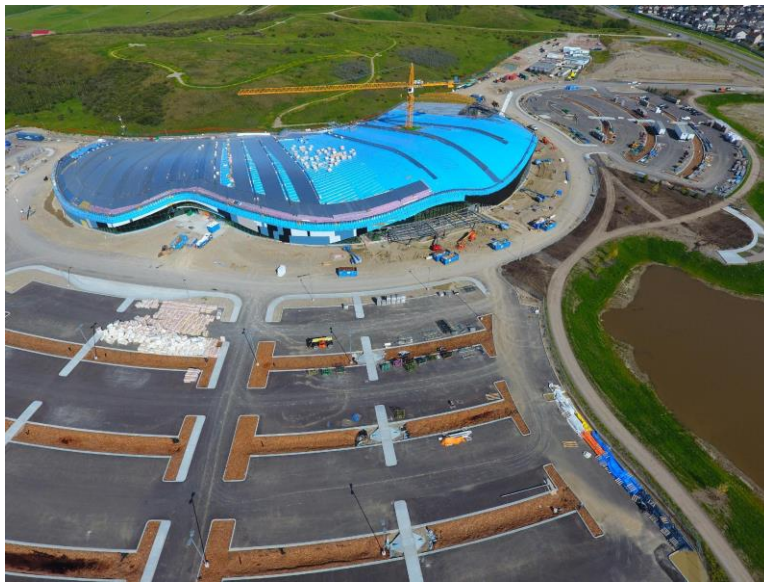
Figure 5. As built image
