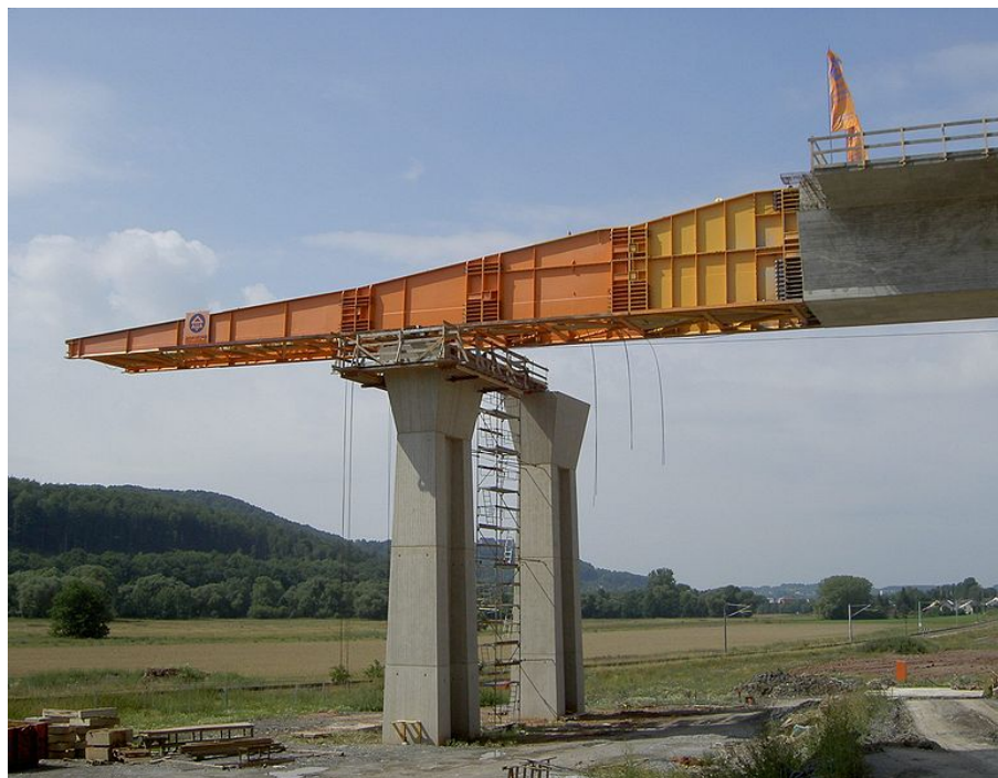
Figure 3: A launching nose of the bridge over the Itz in Germany. Photo by (Storfix, 2005).
