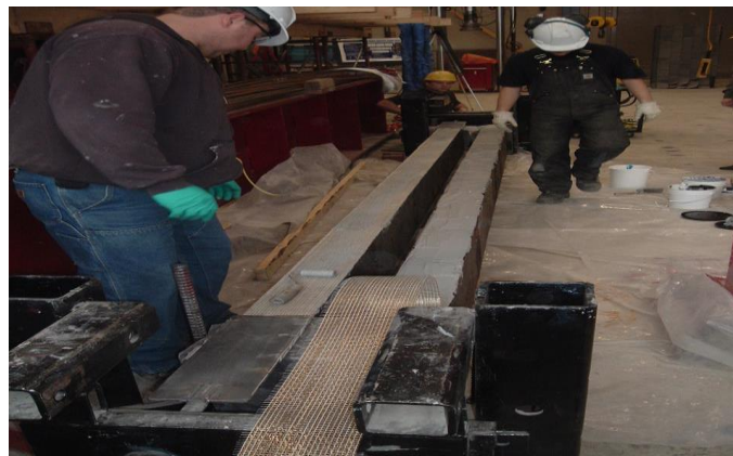
Figure 5: Applying Layer of Epoxy Resin to Bond the Sheet
