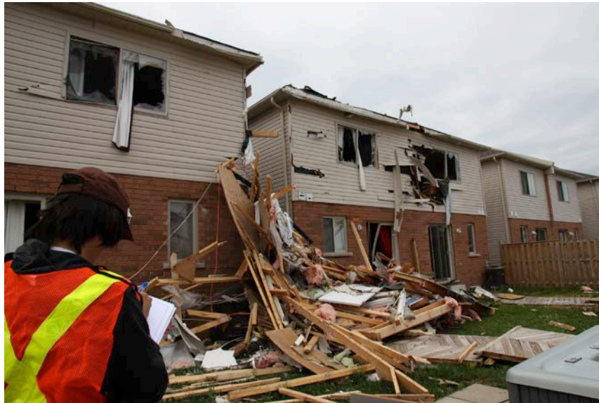
Figure 3. An example of damage caused by debris impacts. This roof had collided with the side of the two houses and as seen in the picture. Many roof trusses are seen in the pile; this roof had blown from a house on Stonemount Cres., across the backyards, ending by impacting these houses on Banting Cres.
