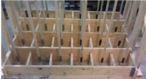
Fig. 3 View of formwork with GFRP bars
