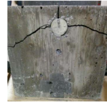
(c) Bar slippage from the anchorage head and concrete cover splitting in case of zero embedment length with bar head in case of #6 GFRP bar (BS-CCS)
