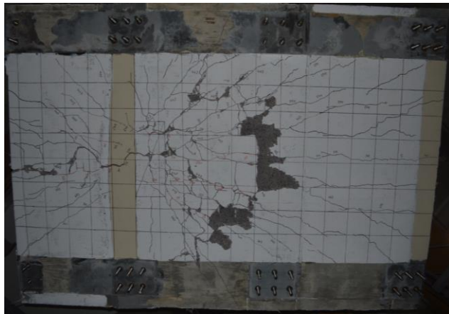
a. Bottom view showing crack pattern
