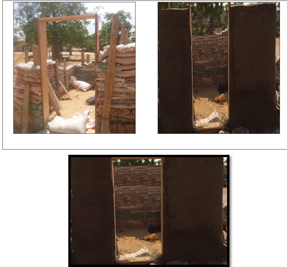
Figure 4: Progress of the Construction of the built Room Model
