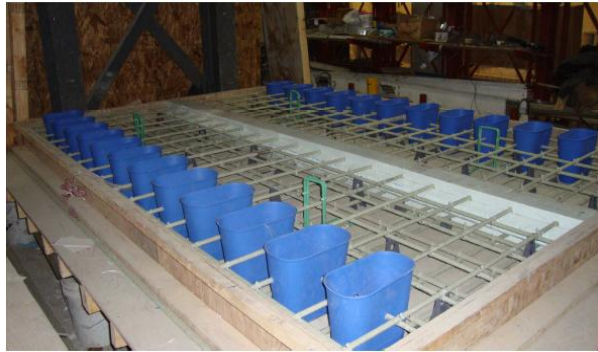
(a) Before pouring concrete
