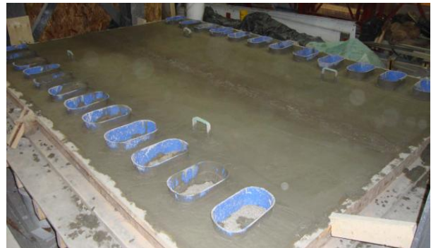
(b) After pouring concrete
