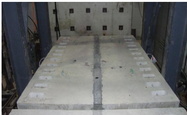
(e) Before grouting
