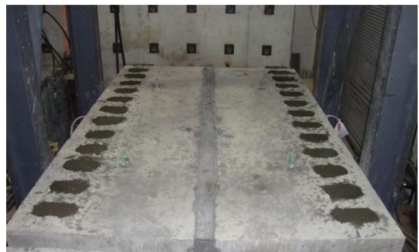
(f) After grouting
