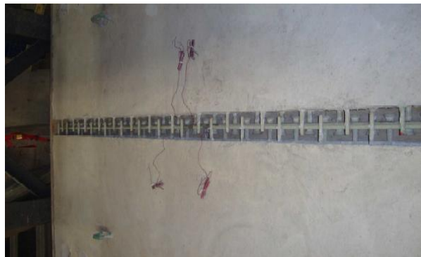
(c) Before pouring UHPC
