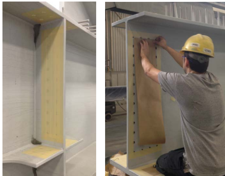
Figure 1: Masking off the faying surfaces in shop
