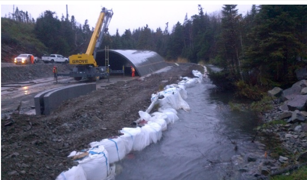
Figure 10. Waterford river diverted to east to permit in the dry construction.
