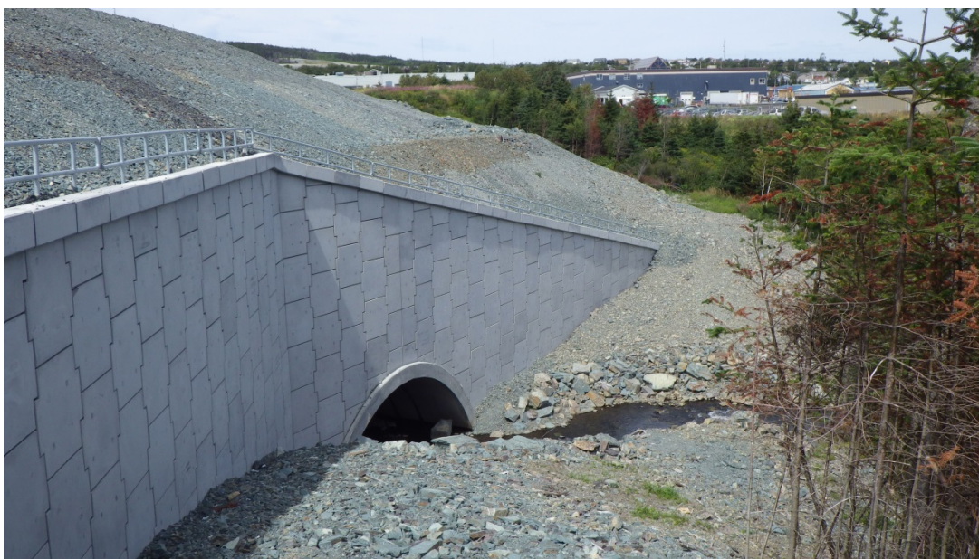
Figure 20. Arch structure complete with head walls, wing walls and embankment.
