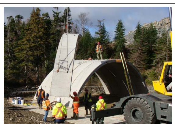
Figure 16. Single crane places elements alternating side to side.
