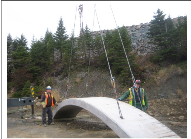
Figure 13. Arch elements are positioned for hoisting and placement.
