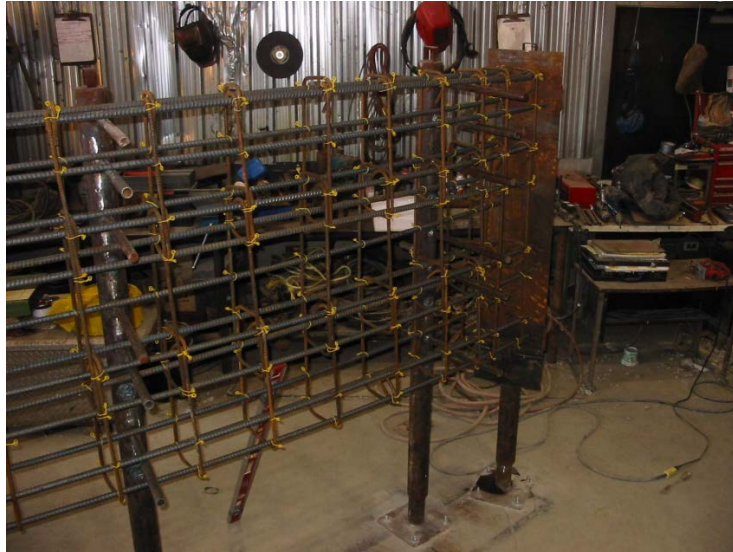
Figure 9. Rebar Cage is assembled on a jig to match archelement curvature
