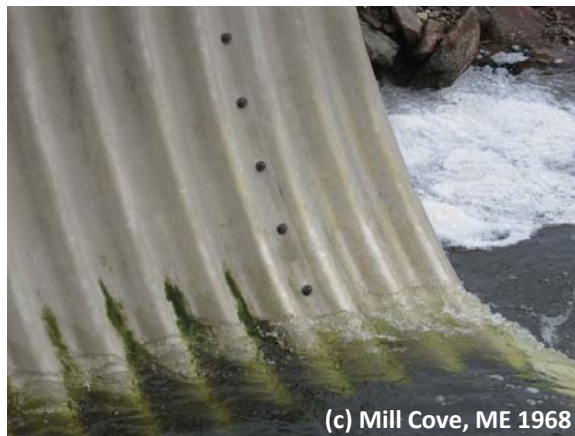
Figure 4: Aluminum structural plate structures in service.
