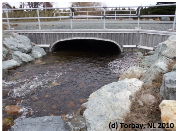
Figure 4: Aluminum structural plate structures in service.
