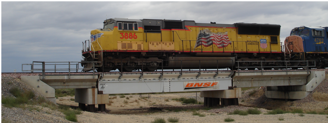
Figure 2.2: Test train crossing 42-foot HCB span at TTCI Pueblo, CO, test facility
