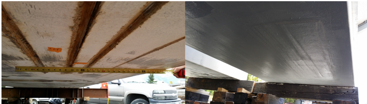
Figure 4.1. Before and after photos of repaired HCB unit
