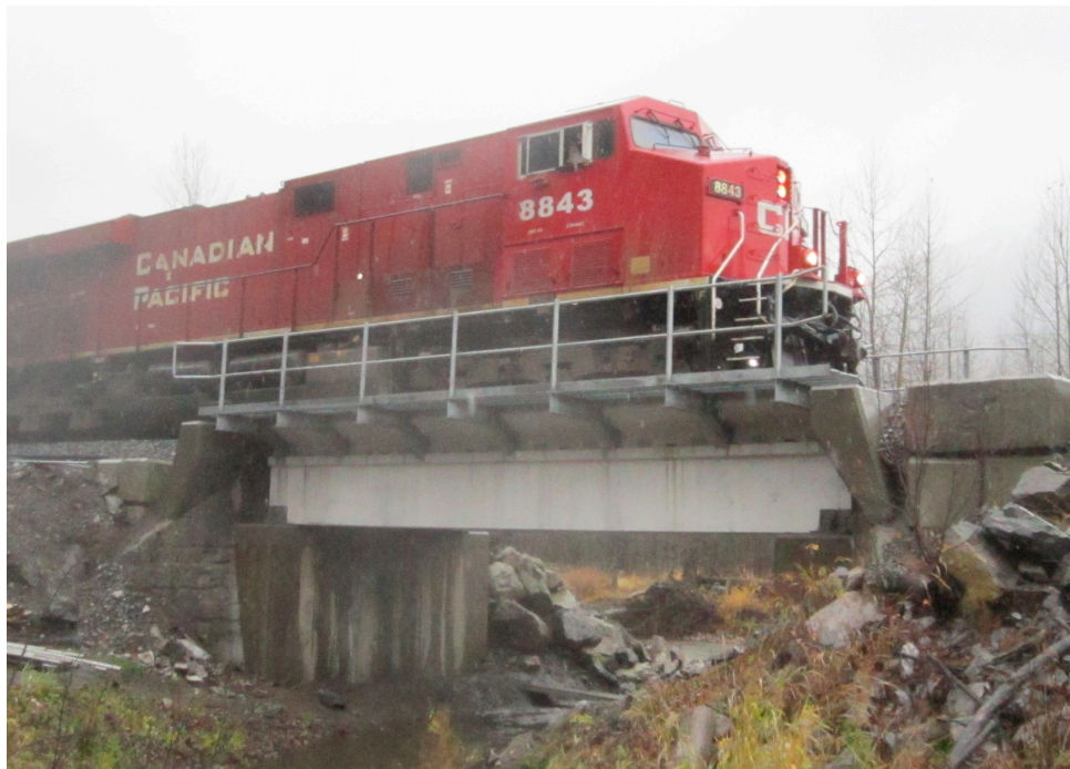
Figure 3.6: Completed installation of the hybrid-composite beam (HCB) span
