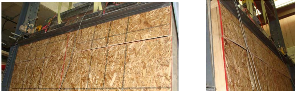
Figure 5. SW-1 Stud wall views after failure showing OSB sheet joint widening near the top of wall
