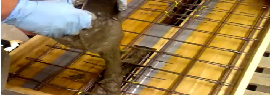
Figure 7: Casting of highly flowable ECC mixture into the mould
