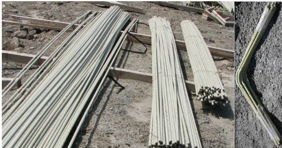
Figure 2: Straight and bent sand-coated GFRP-reinforcing bars as shipped to the site
