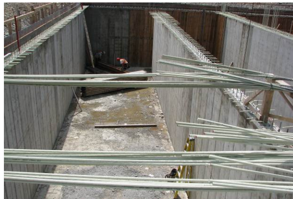
Figure 4: Overview of vertical walls.
