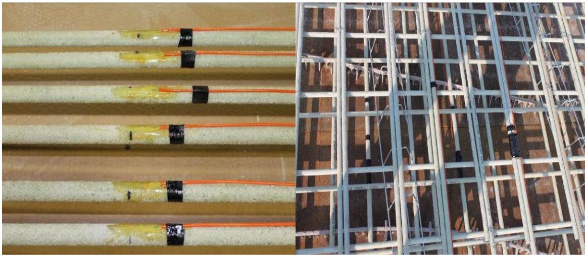
Figure 6: Preparation and instrumentation of GFRP bars
