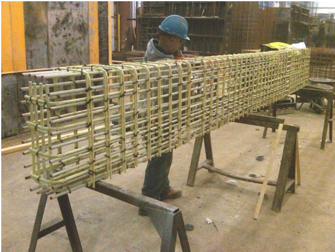
Figure 8: Reinforcement Cage being tied at precast plant
