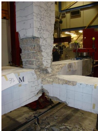
(a) General view of the beam
